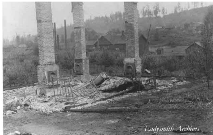
Burned out Residence at Extension Mine, BC (Morden Mine News Sept 2013)
